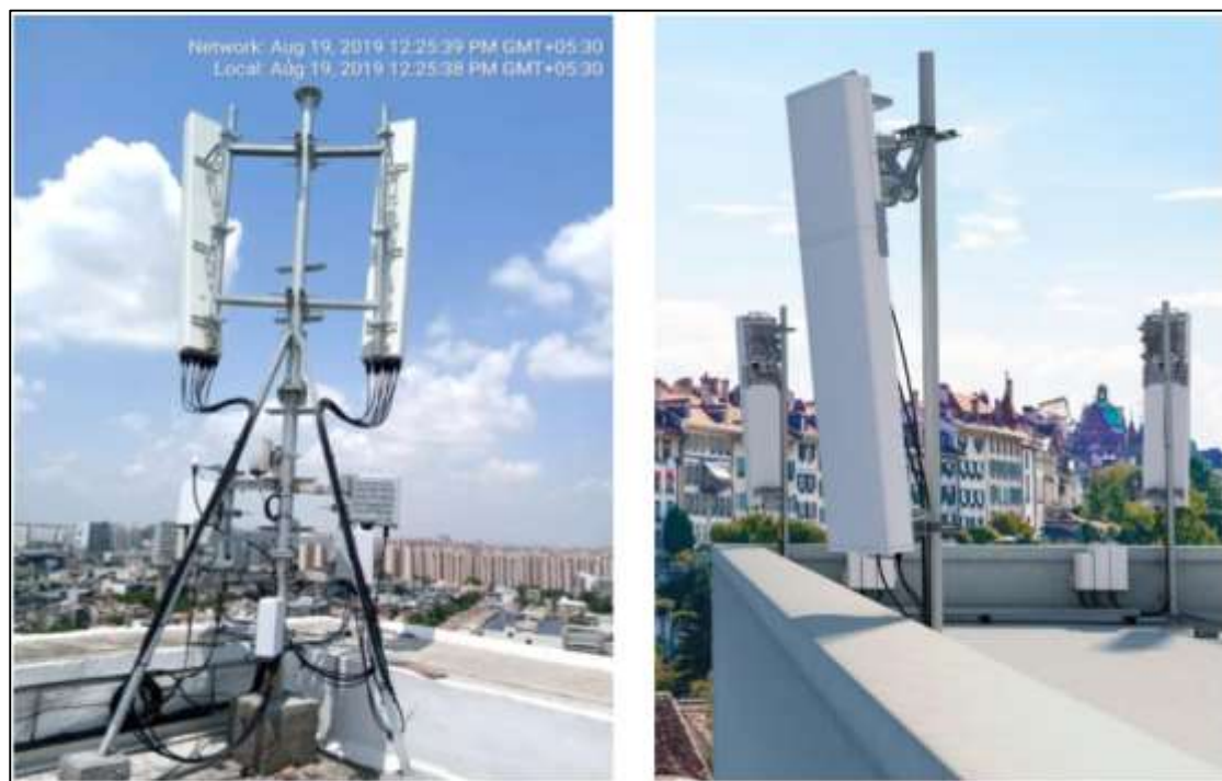
Figure 2. 26: eNB Antenna with RRH (Actual scenario)
