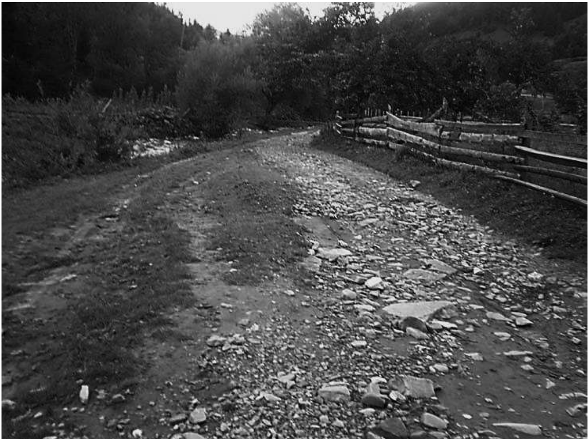
Fig. 3. Use of waste from the stone industry for road pavement
