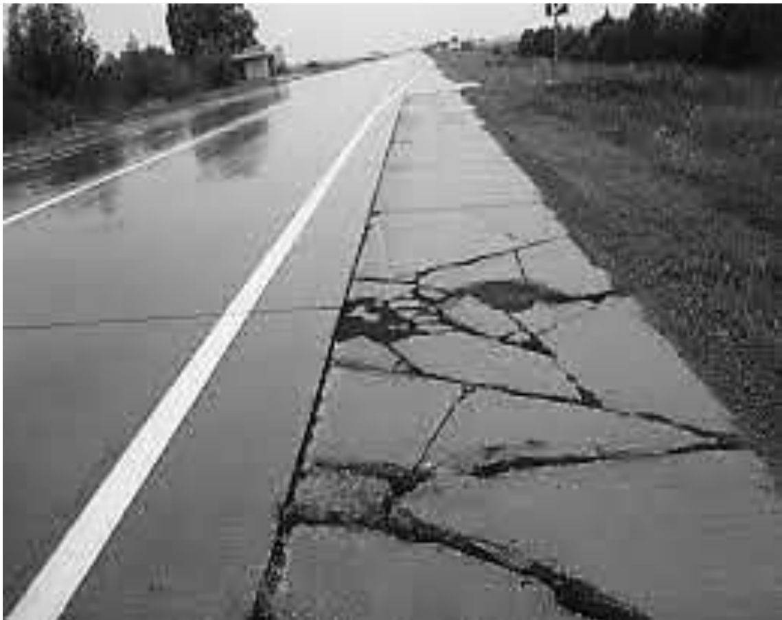
Fig. 9. Road with solid asphalt-concrete coating
