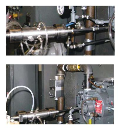
The use of a device with an operating diameter of 25 mm, designed to form an emulsion of diesel 2 and tap water in a ratio of 70% diesel to 30% water in a modern boiler.
