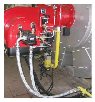
**Figure 1-1 - 2**, - the figure shows an automatic fuel system module for an industrial boiler with a capacity of 10 tonnes of steam per hour.
